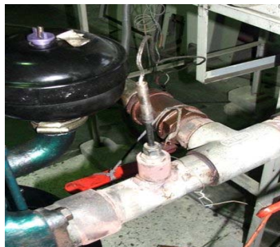
Plate 3.9: Temperature Measurement Arrangement
