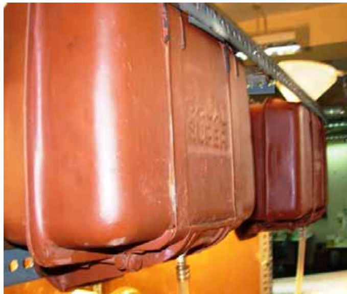
Plate 3.12: Two Tanks System
