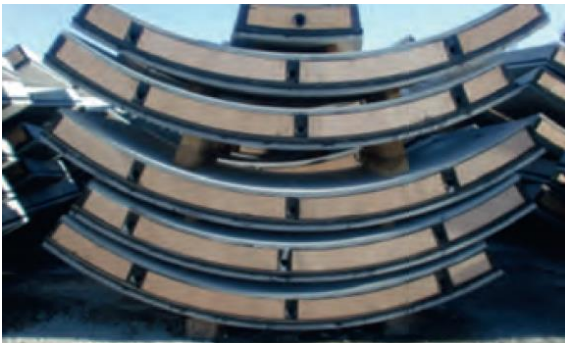
Fig. Segment Stacking for Storage & Transportation
