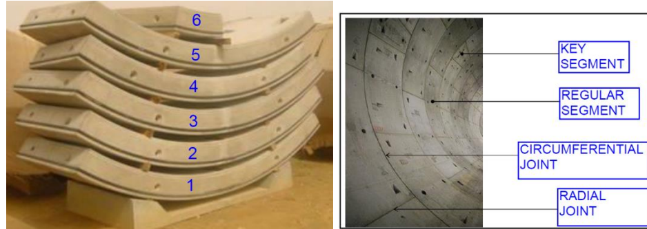
Figure 3.1: Arrangement of Segmental Lining
