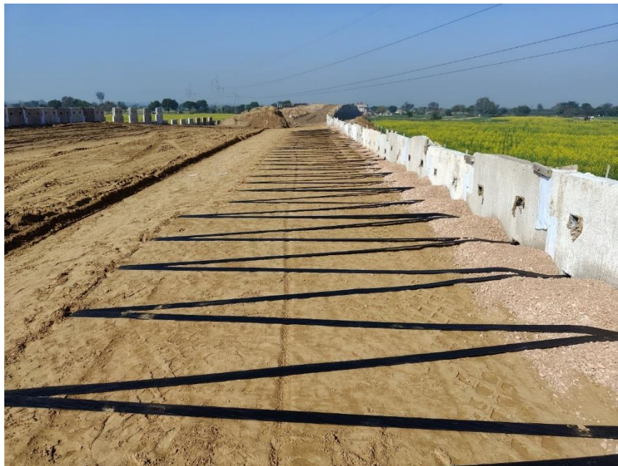
Figure 3.2 Geometry and Site condition of the Reinforced Earth wall at chainage 4+300 to 4+400.
