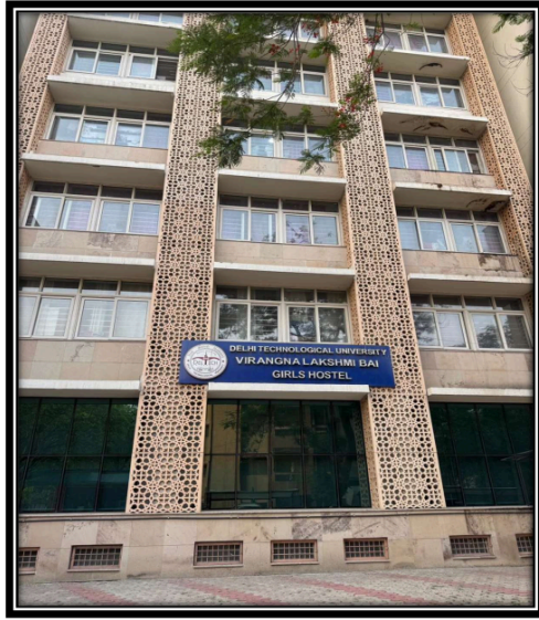
Fig.3.4: AC Hostel (VLB) outer view
