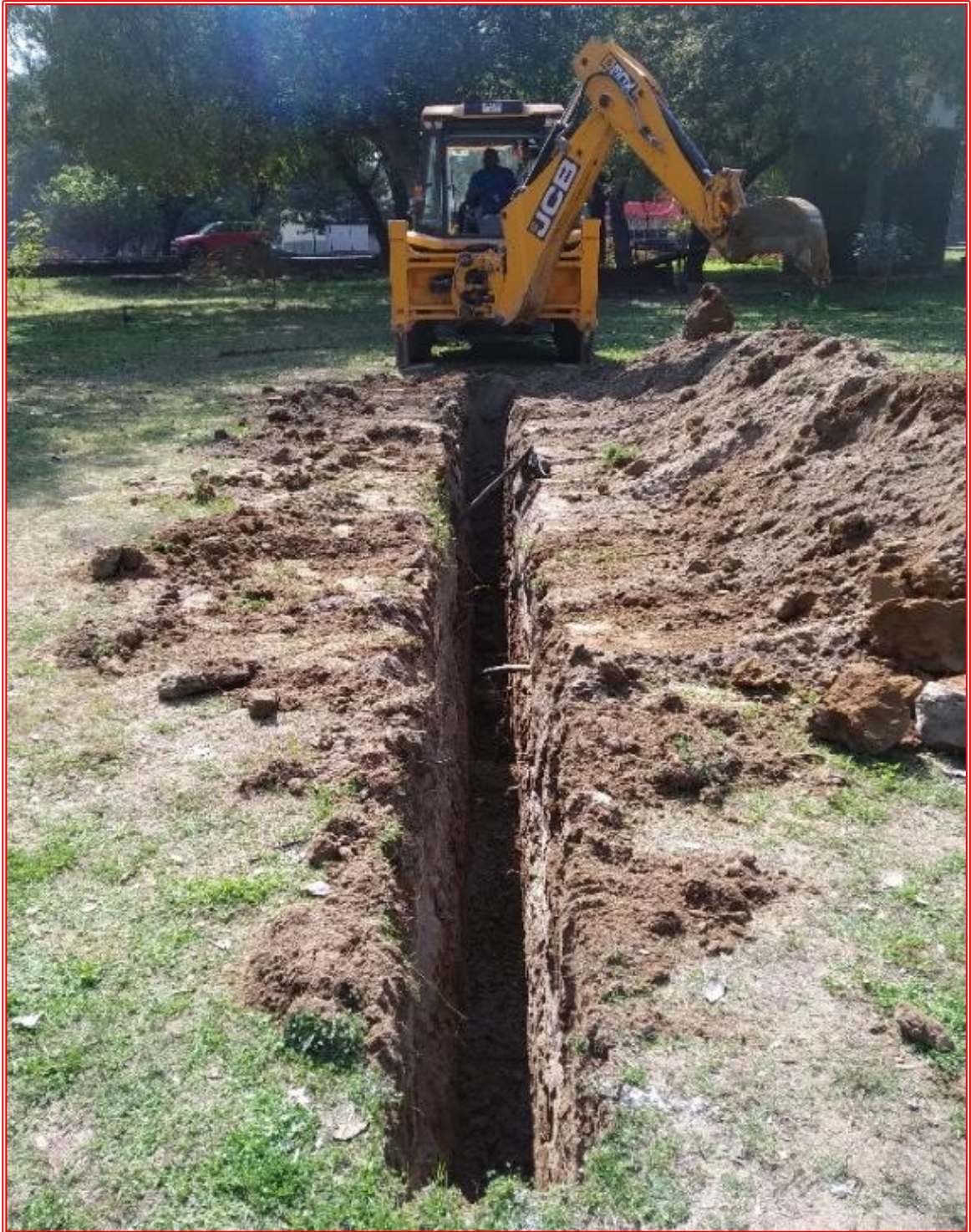
Figure 29: Excavation of wave barrier trench at test site location with JCB excavator
