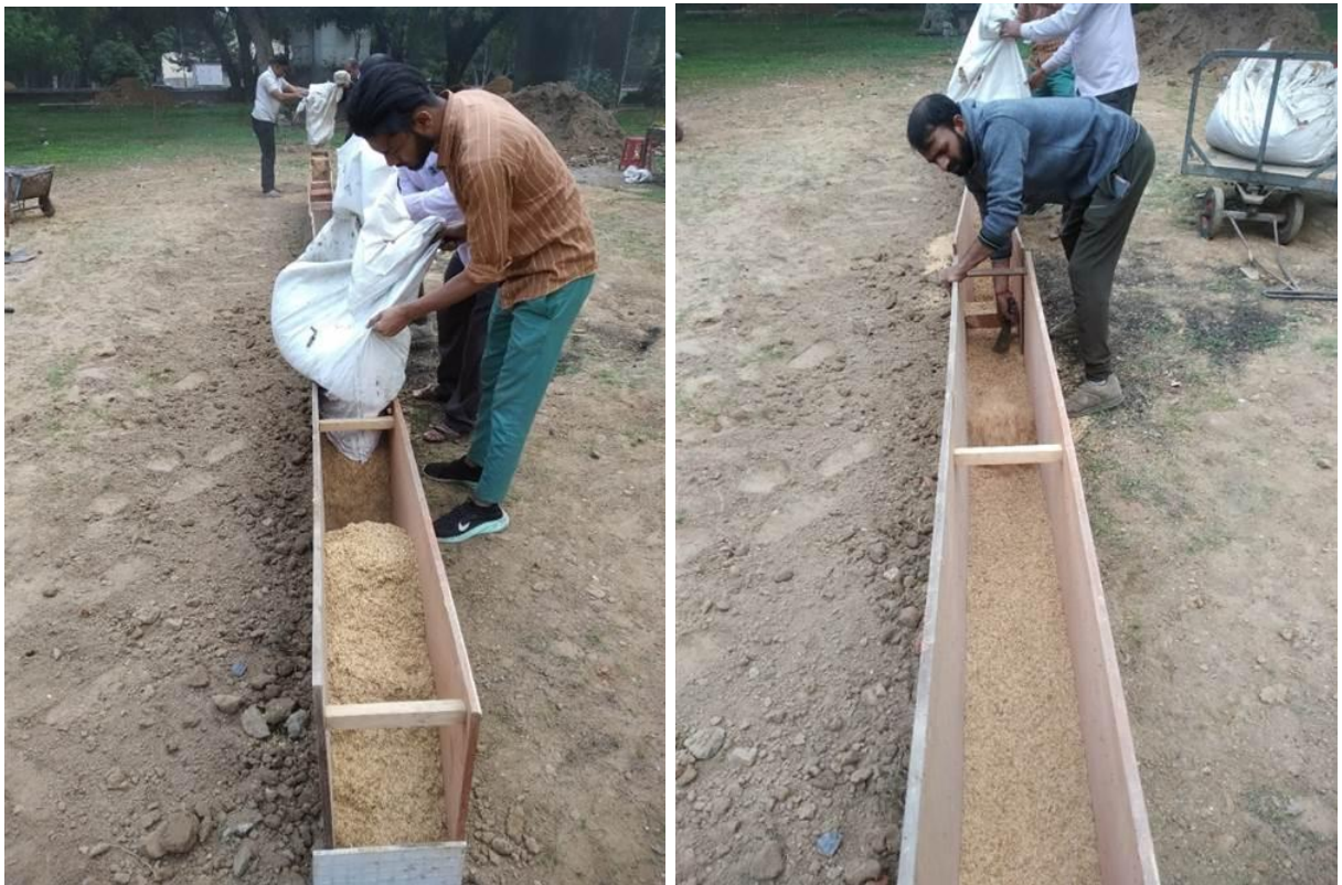
Figure 80: Filling of trench with in-filled material and compaction in progress
