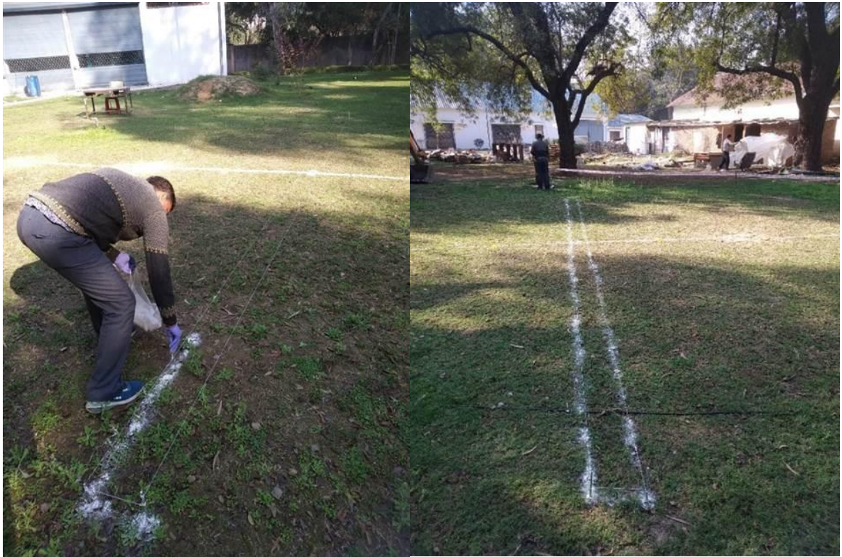
Figure 65: Fixing layout of trench over the ground
