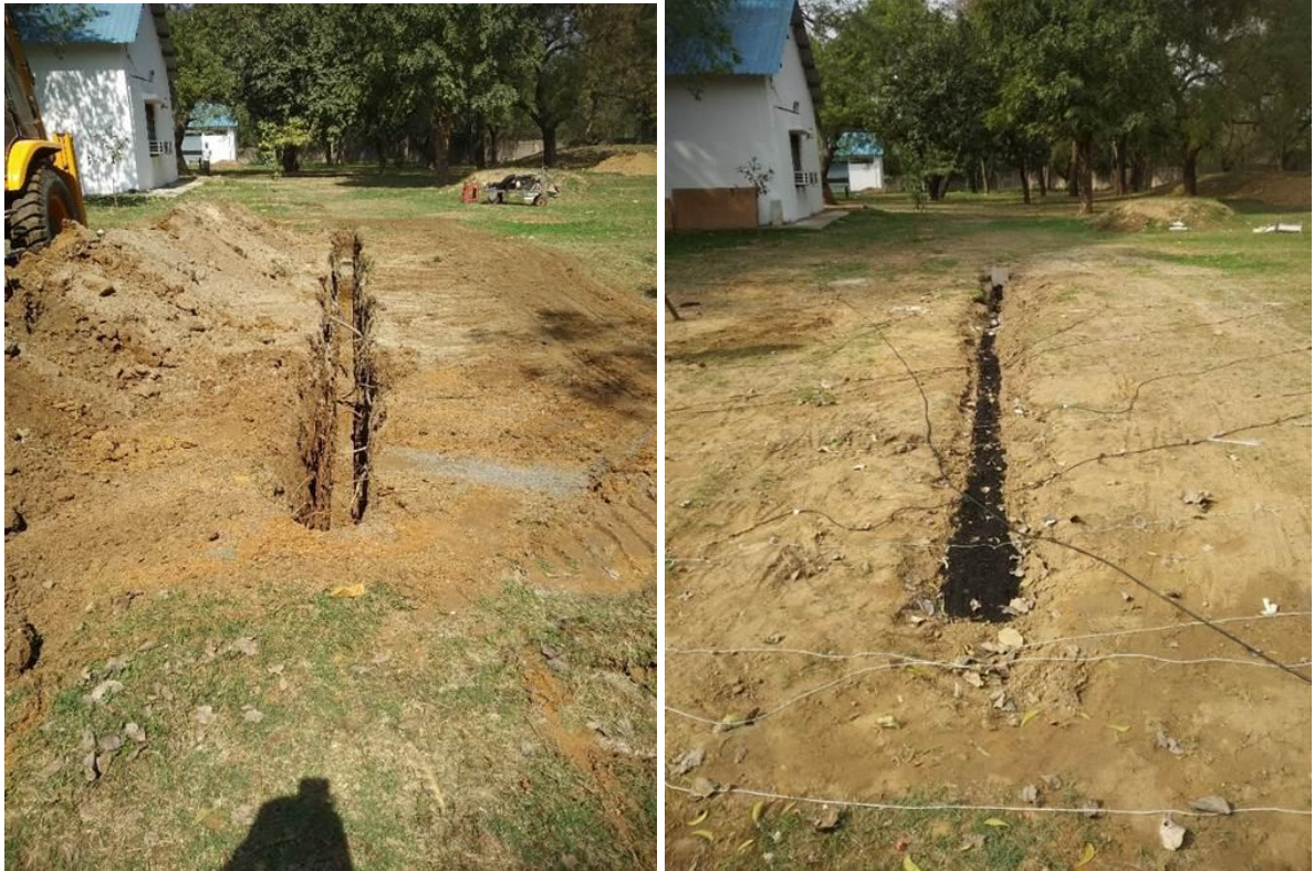
Figure 77: Empty trench and in-filled trench with material Crumbed rubber
