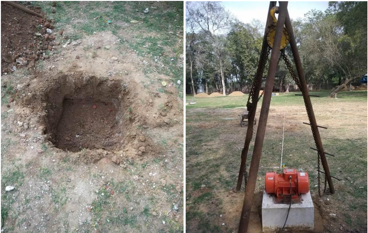
Figure 78: Excavated pit for Oscillator and Oscillator set up with tripod system
