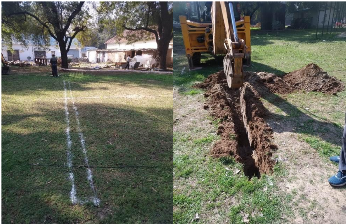
Figure 66: Layout of trench and excavation in progress
