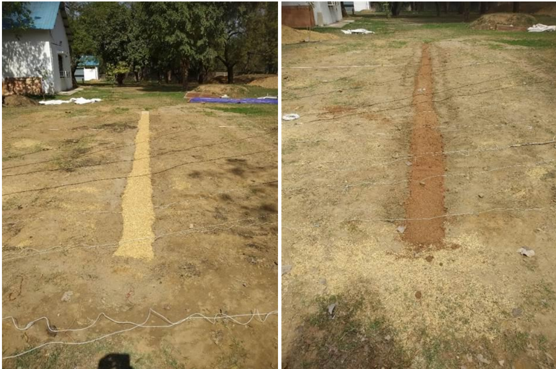
Figure 81: In-filled rectangular trench with materials Rice Husk and Saw dust
