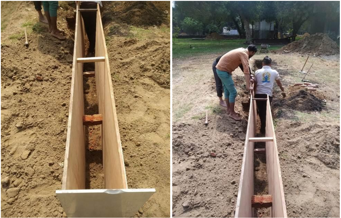
Figure 79: Filling of trench with in-filled material and compaction in progress
