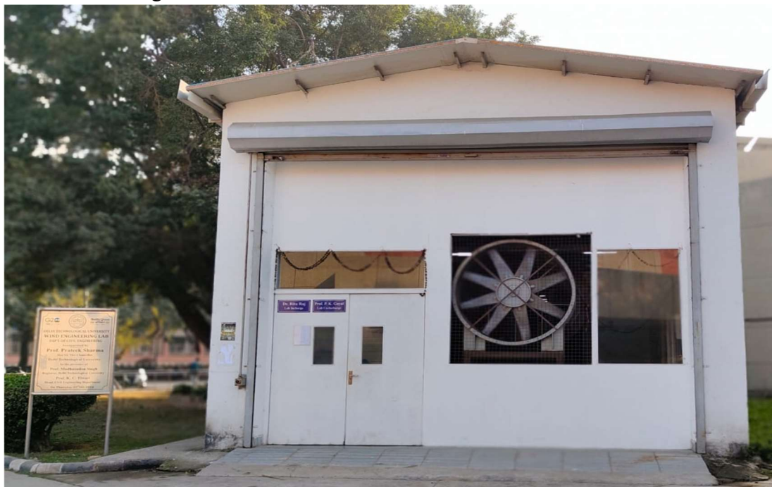
Fig.3.1: Wind Engineering Laboratory at Delhi Technological University
