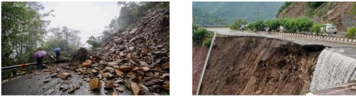
Fig 1. Landslide event, slope failures in Shimla region
