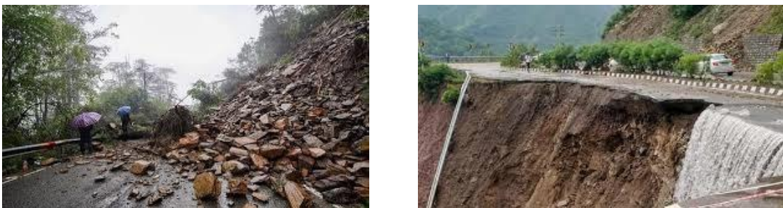
Fig 1. Landslide event, slope failures in Shimla region
