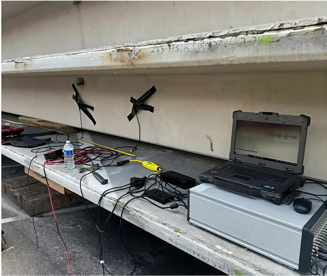
Figure 4.1: Experimental reinforced concrete setup with piezoelectric sensor placement
