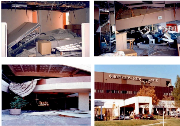
Figure 1.2 Failure of office partitions, ceilings, light fixtures, heavy soffit and HVAC.
