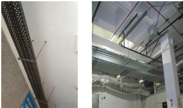
Figure 1.1 Non-Structural Components in a building
