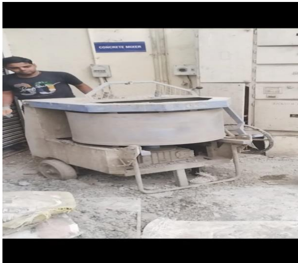
FIGURE: 4 CONCRTE MIXING
