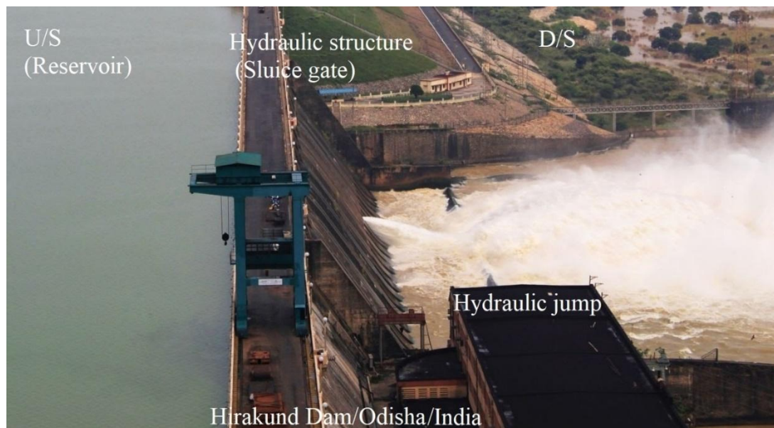
Figure 1.2 Phenomenon of hydraulic jump occurring downstream of the Hira Kund dam, Odisha, India
