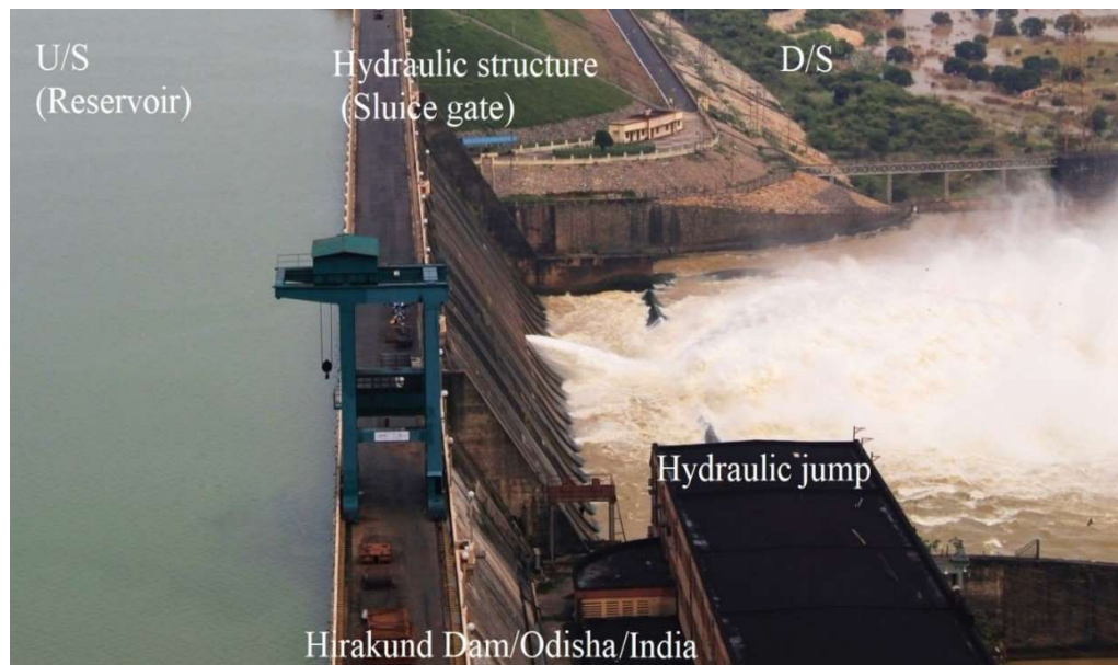
Figure 1.2 Phenomenon of hydraulic jump occurring downstream of the Hira Kund dam, Odisha, India
