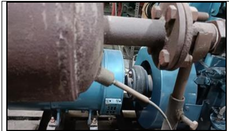
Plate 3.15 K-Type Thermocouple
