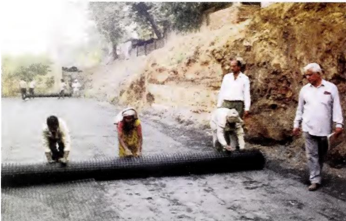
Figure 1.3 Spreading Geogrid as Basal Reinforcement at Okhla [1]
