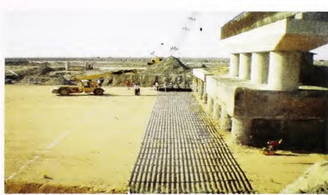
Figure 1.6 Installation of Bonded Geogrid, Mundra, Gujarat
