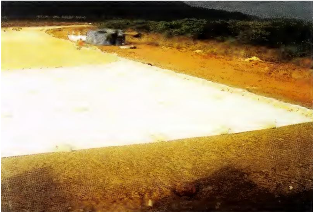
Figure 1.5 Geotextile as Basal Reinforcement at Visakhapatnam
