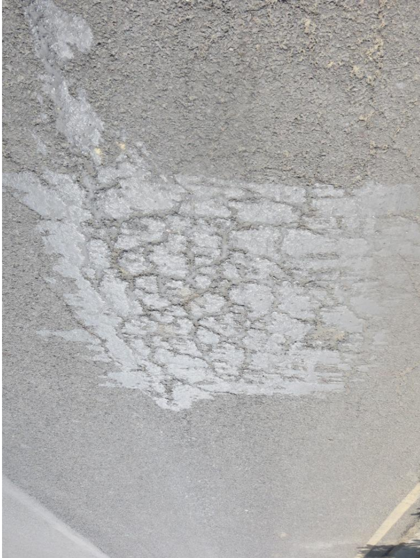
Photo -5.12 Map cracking of pavement
