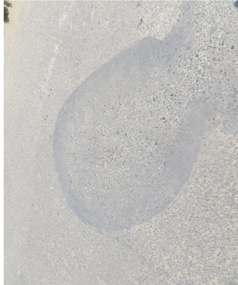
Photo – 5.9 a & b Repaired pot holes of pavement surface
