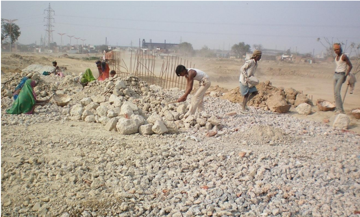
Photo-3.3 Manual crushing of demolition waste
