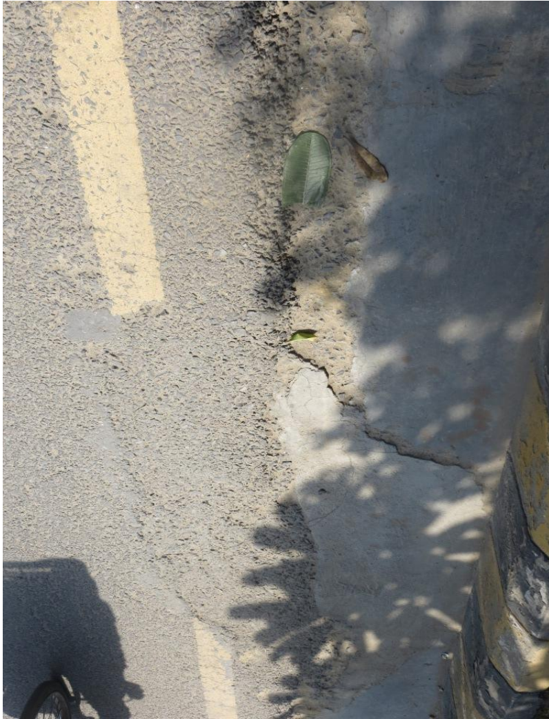
Photo 5.10 Repair at edge Pavement defect
