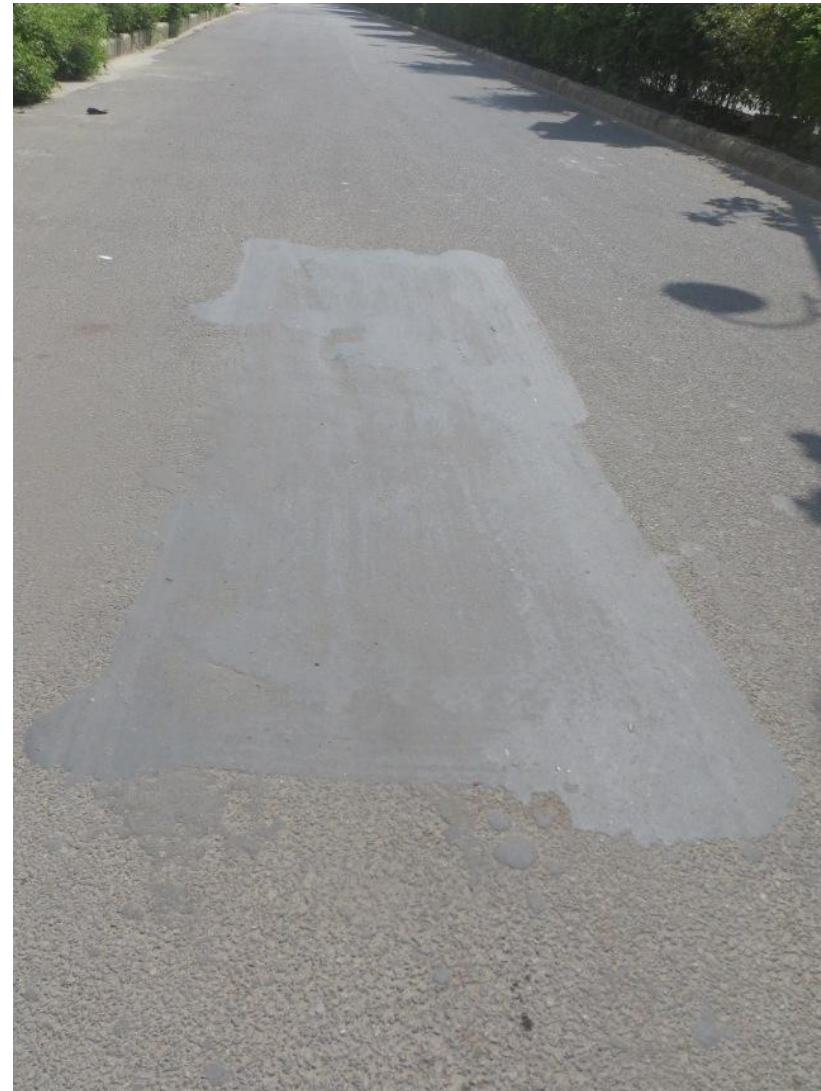
Photo -5.13 Pavement surface after repair of map cracking
