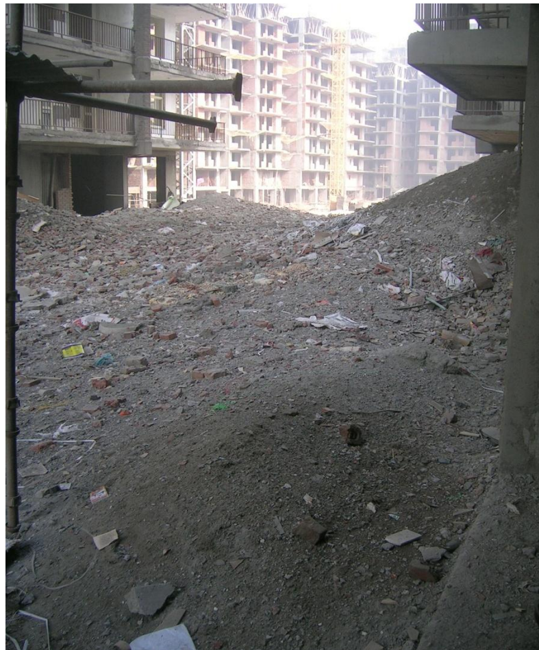
Photo-3.6 Sampling of mortar and masonry waste of a construction site
