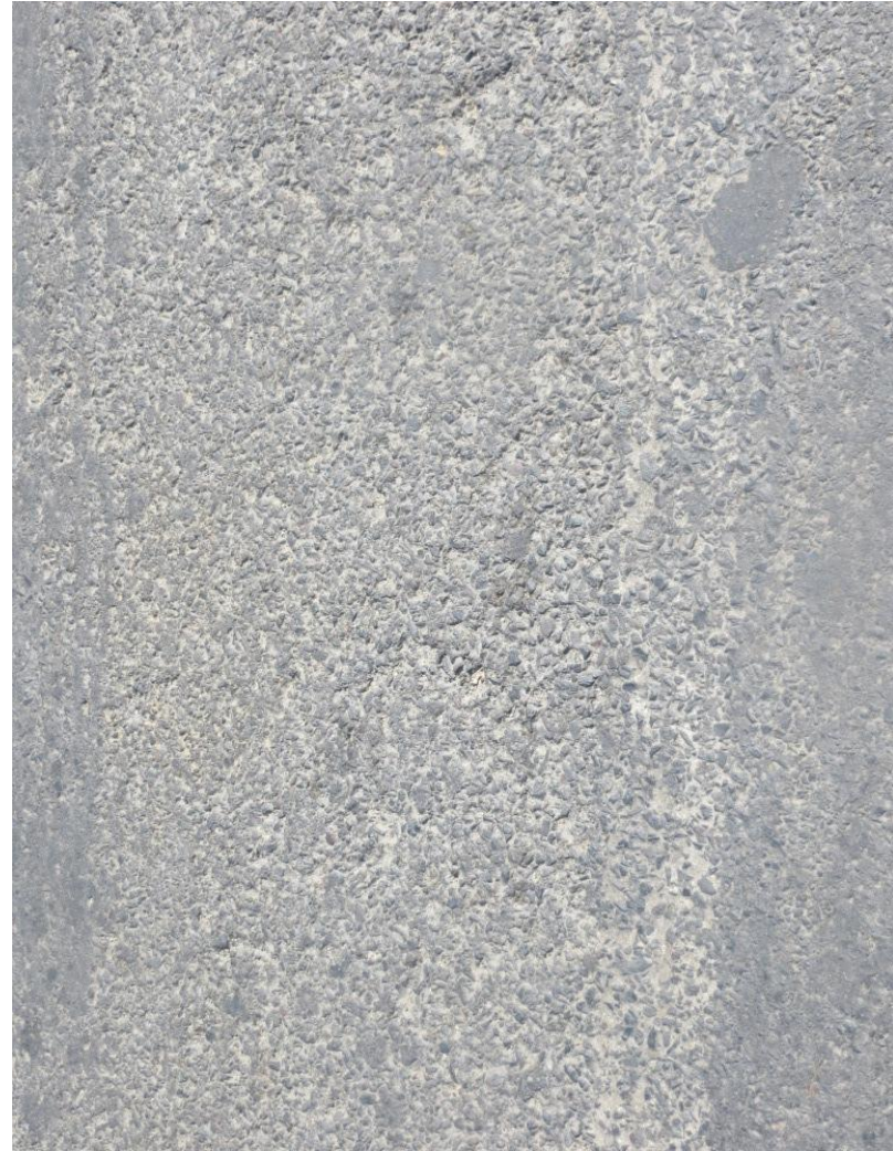
Photo 5.11 Chipping of aggregates from top surface course
