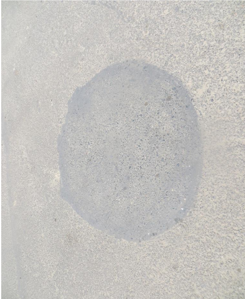
Photo – 5.9 a & b Repaired pot holes of pavement surface
