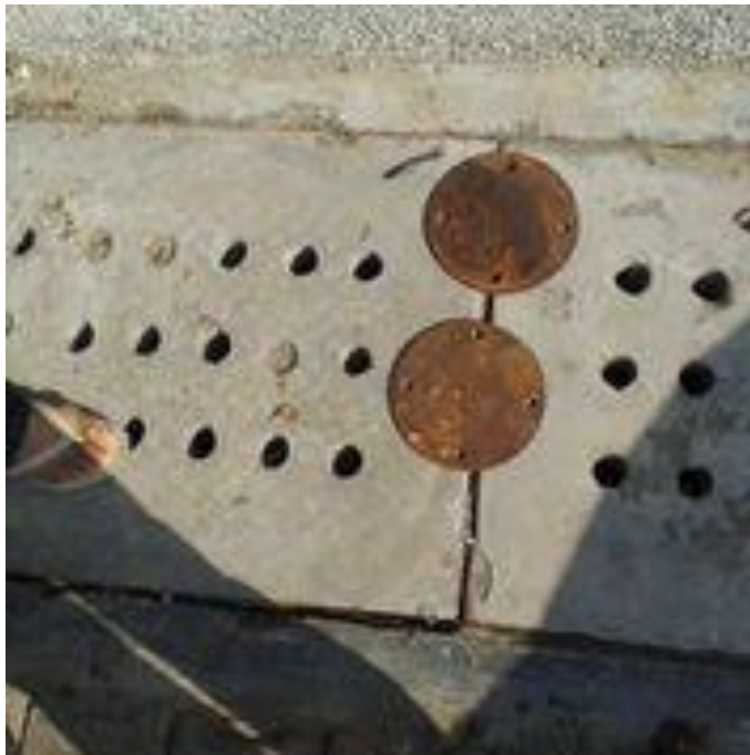
Photograph 14: Cover plate for pile cap.
