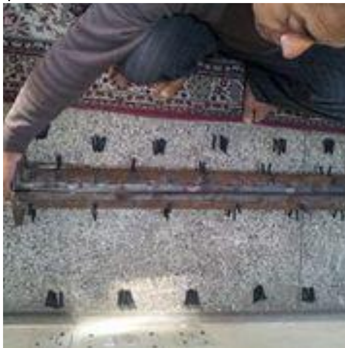
Photograph 18: Zig - zag spikes arrangement (Vertical) (not a part of this thesis).(view 3)
