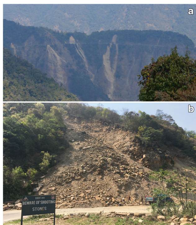
Fig. 1 Panoramic (a) and close view (b) of landslides that occurred on the Phuentsholing–Thimphu highway in Chukha Dzongkhag after the 2016 monsoon
