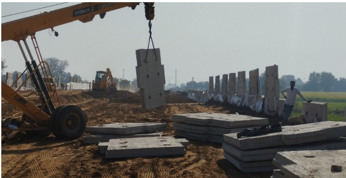
Figure 3.3 Erection of RE Panel
