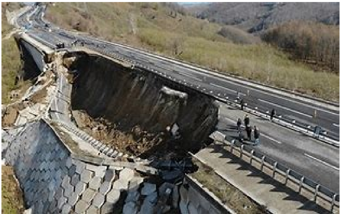
Figure 1.1 Turkey catastrophic RE Wall failure (2021) (AGU Blogsphere) [1]
