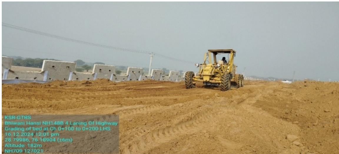
Figure 3.5 Grading of Embankment
