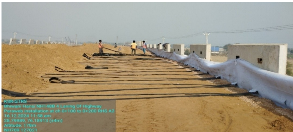
Figure 3.4 Geostrip Installation
