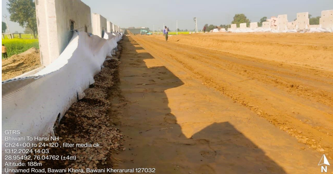
Figure 3.2 Reinforced Earth Wall at Chainage 24+200
