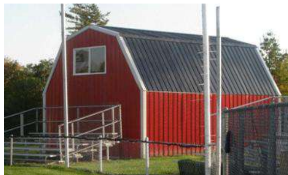
Fig. 1.13: MI Gambrel Roof https://www.hansenpolebuildings.com/
