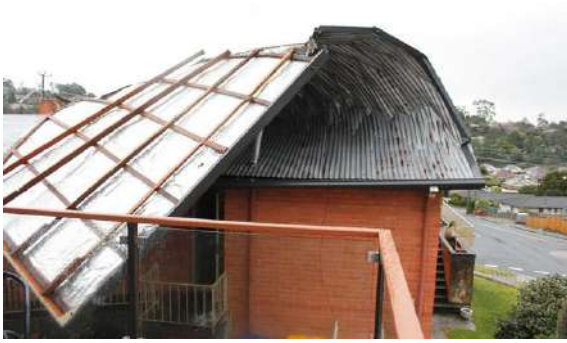
Fig. 1.18: Roof Damage of new building due to wind storm in Tasmania, April 2017 http://www.abc.net.au/news/2017-04-27/the-roof-peeled-back-from-a-house-in-kingsmeadows/8475332
