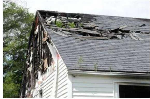
Fig. 1.19: Roof damage of gable roof building caused by heavy winds in Chicago, April 2016 http://www.skylinenewspaper.com/wind-storm-rips-roof-from-apartment-building/
