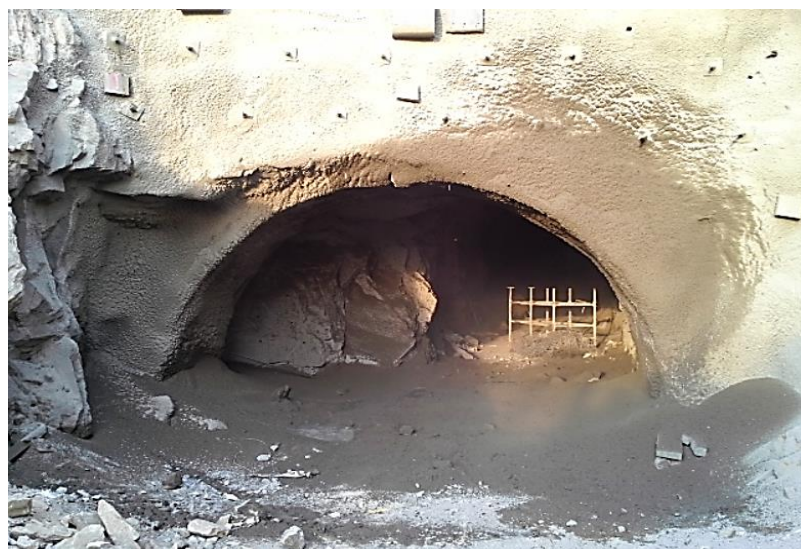
Figure 2.3: Tunnel portal stabilization
