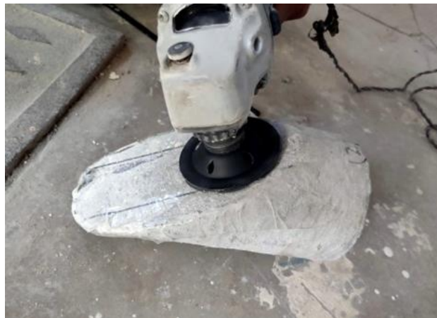
Fig. 4.9 Grinding operation done on the inclined concrete surface
