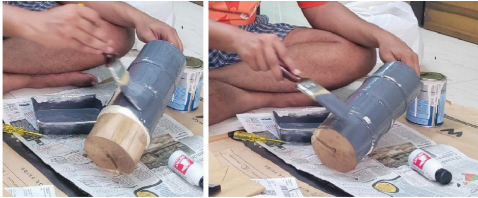
Figure 8.39 Applying primer over wooden surface
