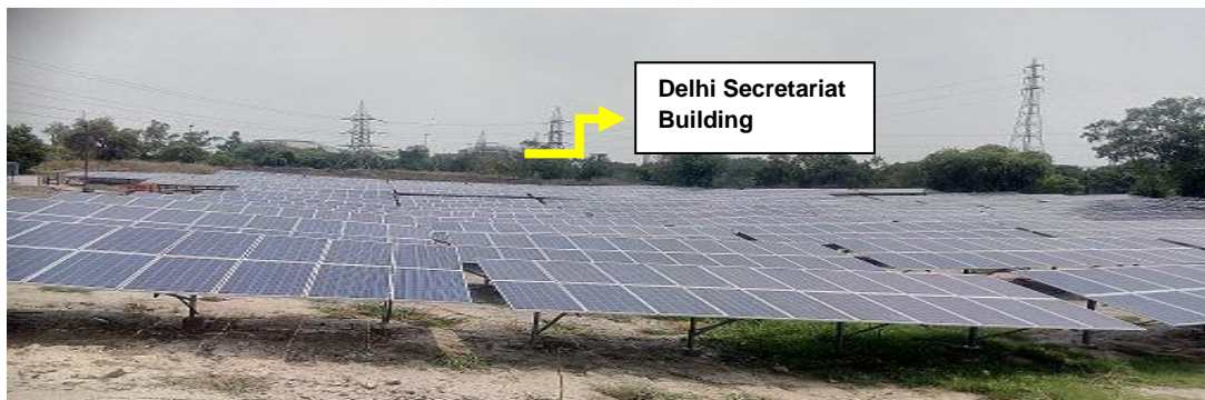
Fig. 4.2 Aerial View of the Solar PV Plant with Delhi Secretariat Building in Background
