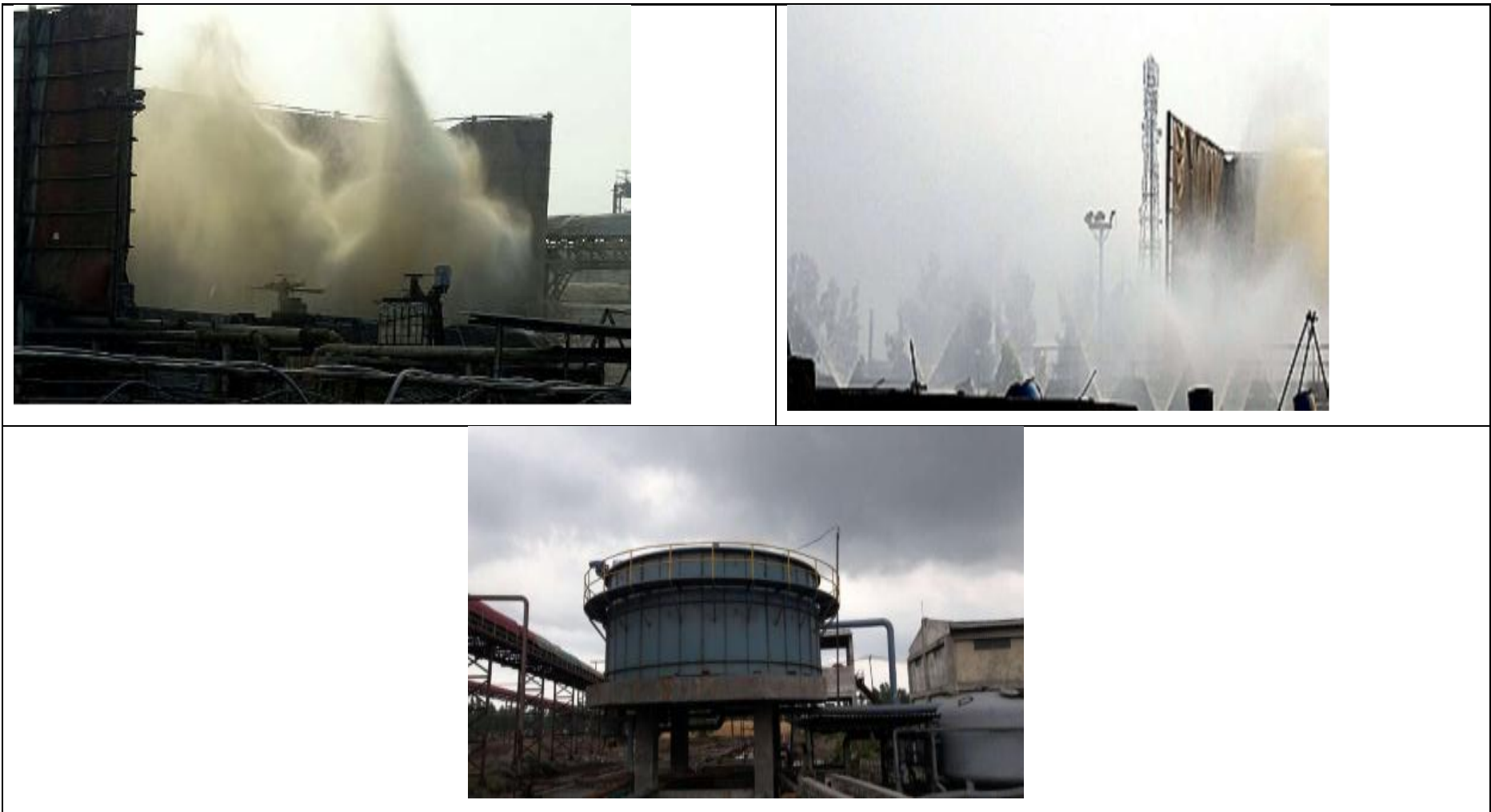
Figure 4.2: ETP at Bindal Paper Mills Ltd
