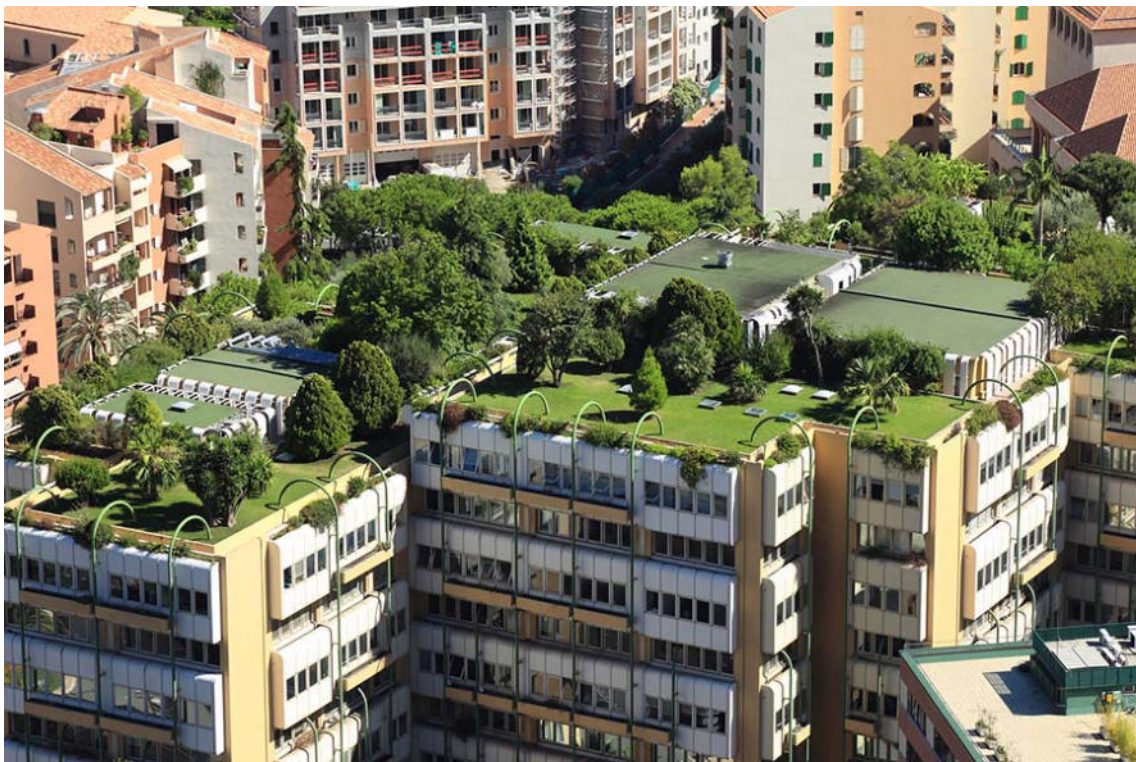
Figure 2.8: Vegetated Roof as LID
