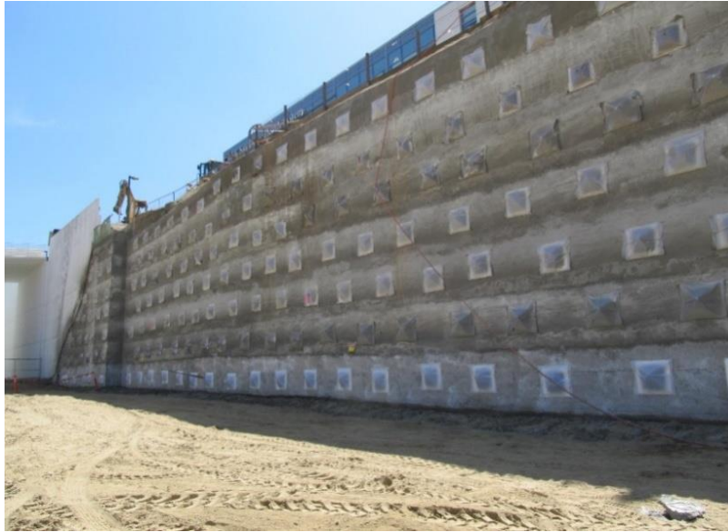
Figure 1.1. Soil nailing (Raju 1996)
