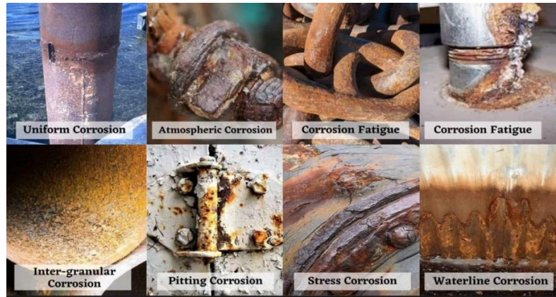
Figure 1.30: Example of corrosion[79]
