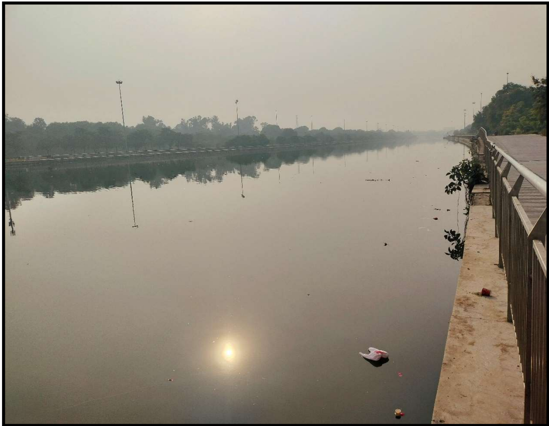
S6 - Upstream Barrage
