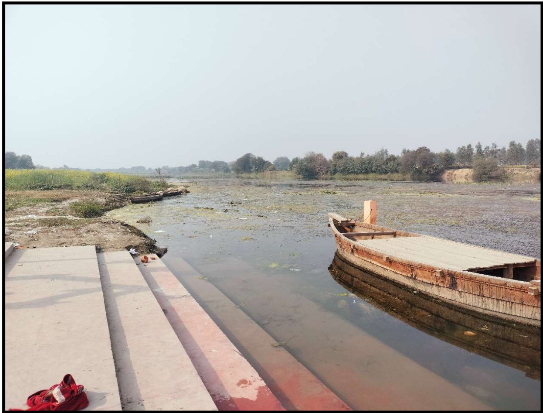
S2 - Up Stream water intake
