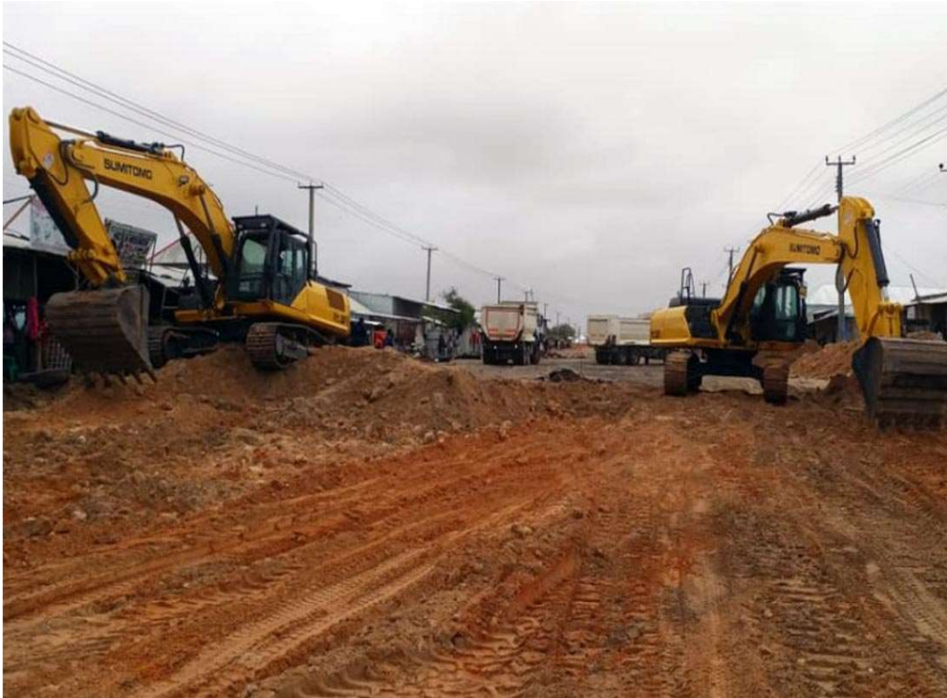
Figure 19 Road construction project in Wadajir district of magadishu
