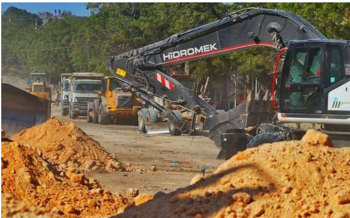
Figure 18 Road construction project in Wadajir District of Mogadishu
