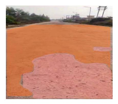
Fig 3.4 Segmentation Example of Road and Pothole
