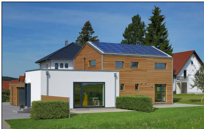
Figure 2.3 Plus energy house Wriedt, Unterallgäu, Germany (Baufritz, 2022)
