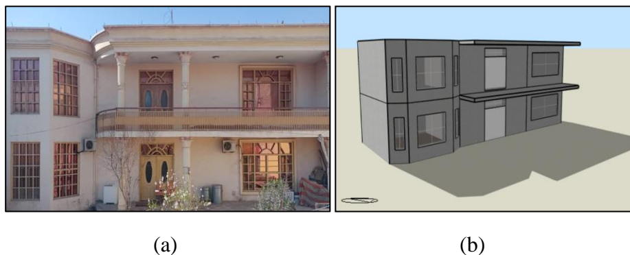
Figure 5.15 Case study building front view a) real-time photography, b) 3D view
