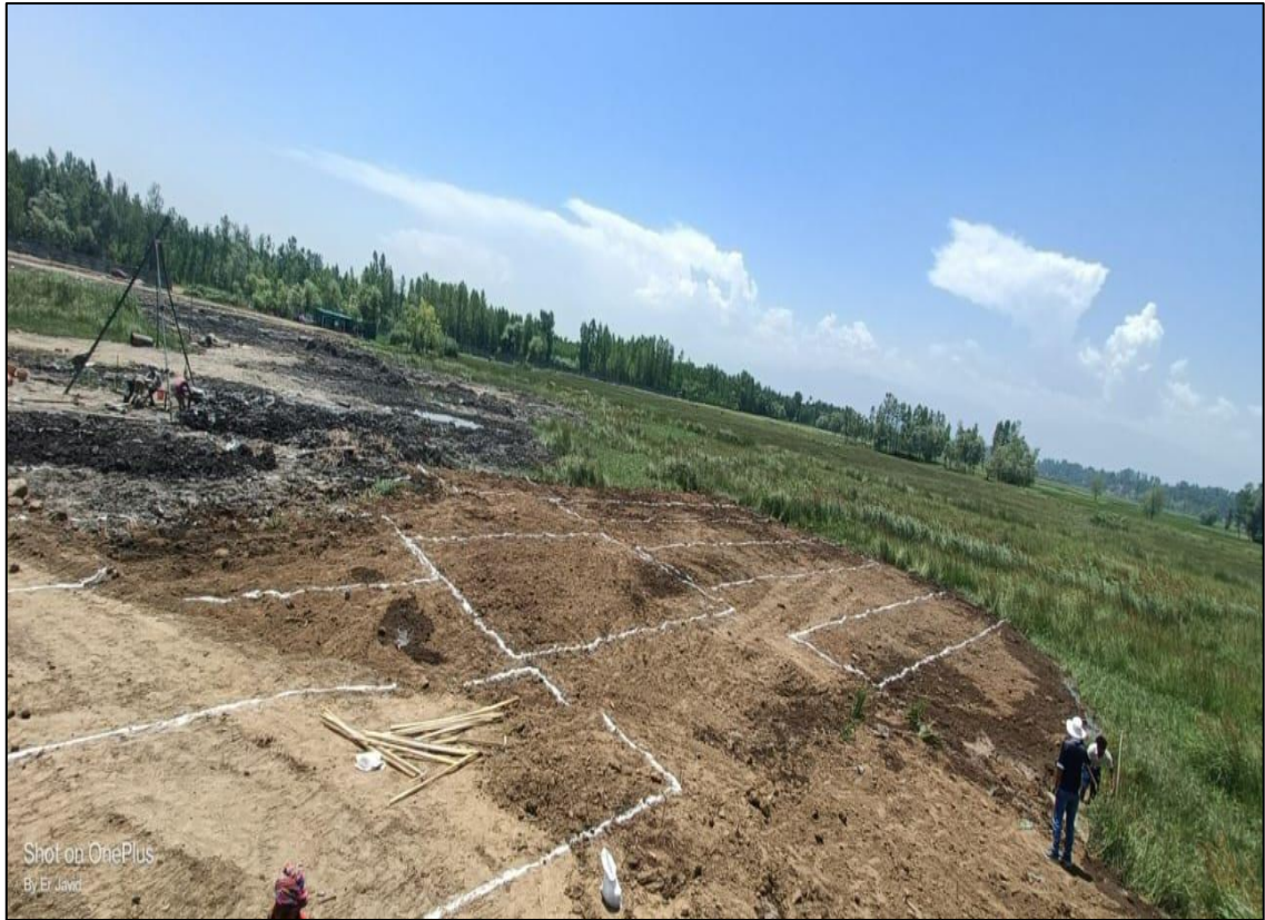
Figure 7 Markings for Triangular Arrangement of Stone Columns at the Site
