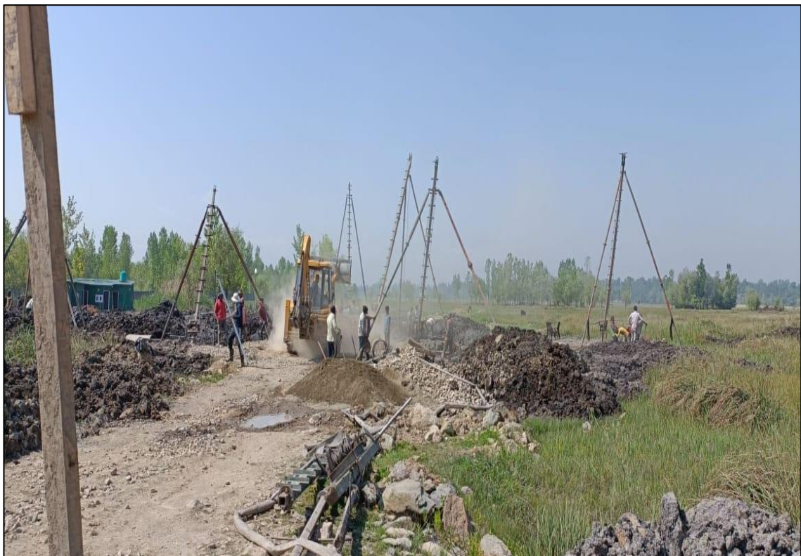
Figure 8 Installing the Stone Columns
