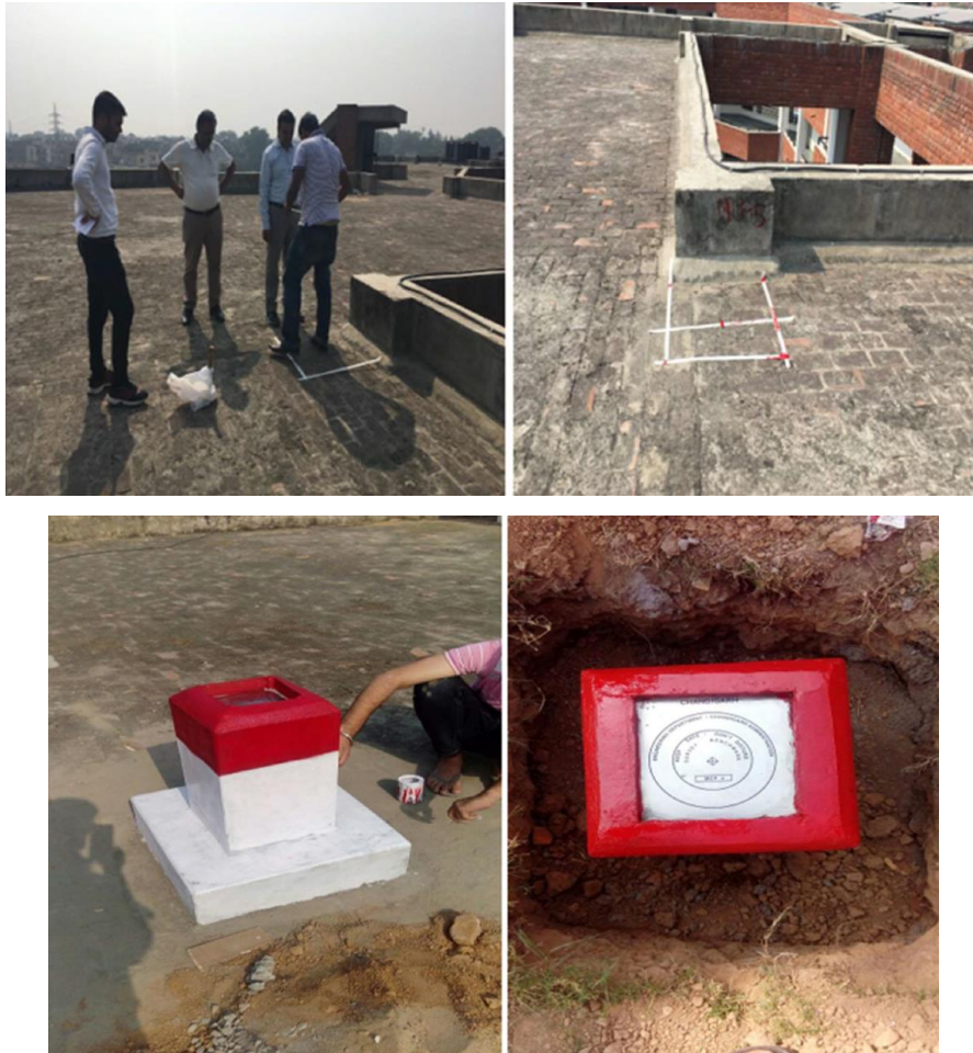
Figure: 37: Survey Monumentation
