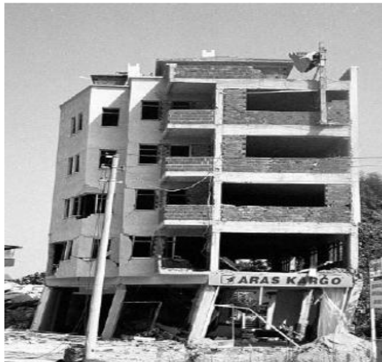
Figure 1.2 Buildings failure due to soft storey [5]
