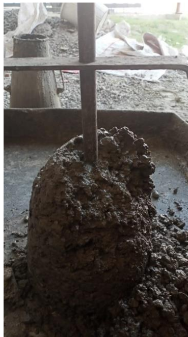
Fig. 4.5 Conducting a slump test on CM
