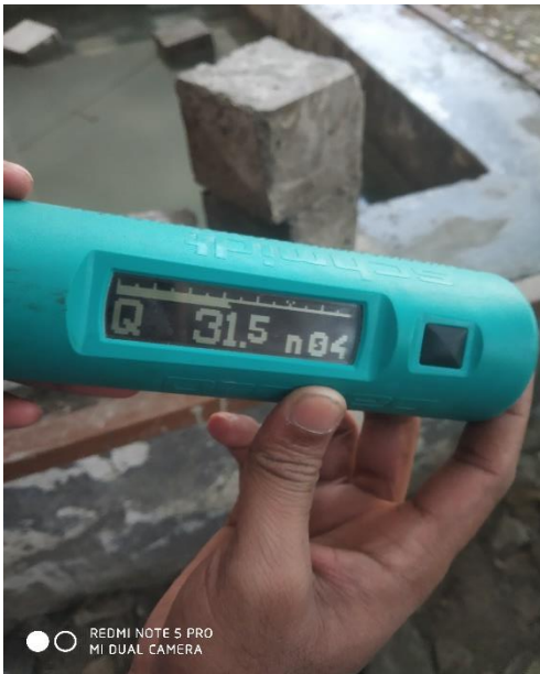
Fig 4.14 Rebound hammer Reading 4
