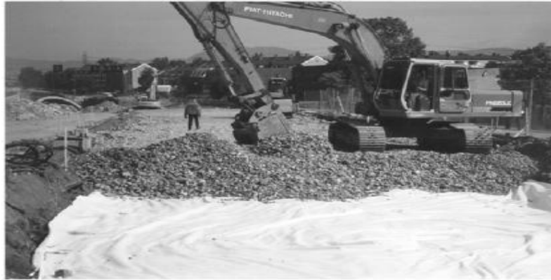
Fig 1.13: Recycled Aggregate used as Granular Base Course
