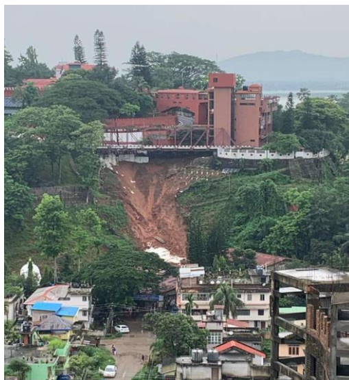
Figure 3-1 Landslide at Raj Bhavan, Guwahati Assam
