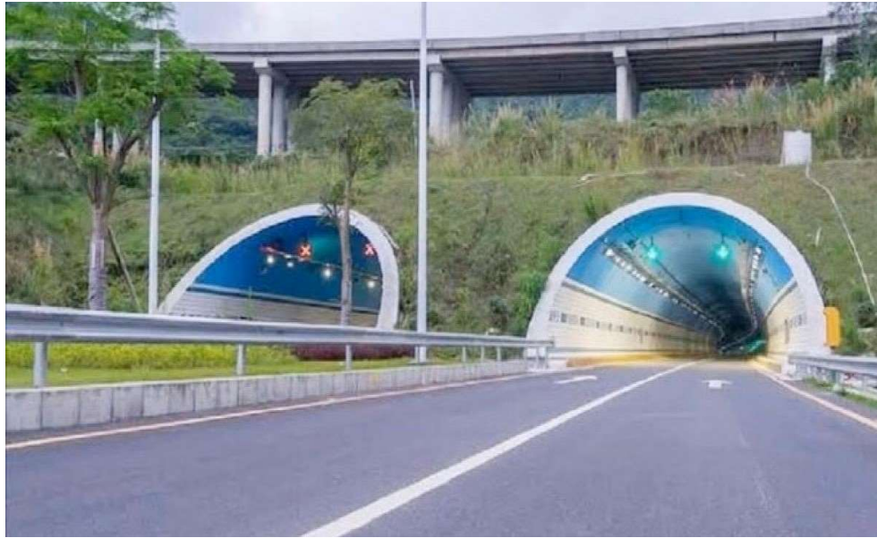
Fig. 1.2 Thane-Borivali Twin Tunnel. (Source: Swarajyamag.com/Thane Borivali twin tunnel )
