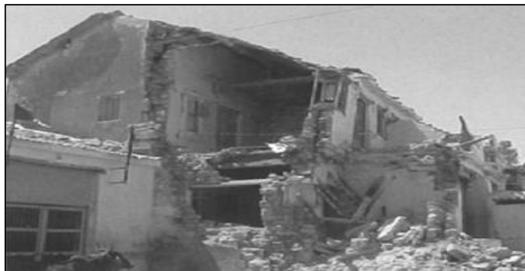
Figure 16: Due to the lack of through-stones and the use of thick walls made of small rubble, the walls often split into two layers, which compromised their ability to bear gravity loads.
