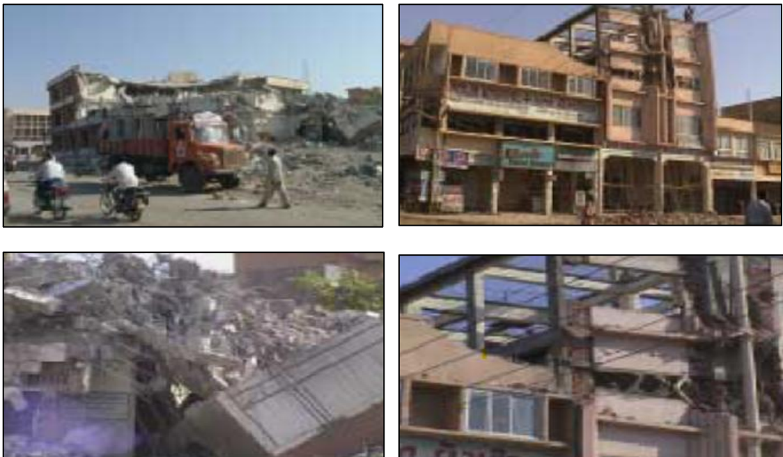
Figure 52: Manual demolition and removal of wreckage of damaged hospital building with mid-floor collapse in gandhidham. wreckage showing showing clear separation of concrete and steel.(RCC) and indicated the quality of material.
