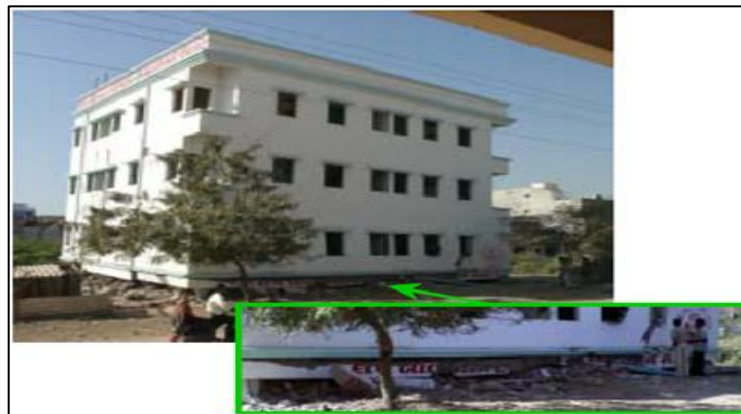
Figure 51: The collapsed ground floor of the children's hospital and research center in Gandhidham is a typical example of soft ground floor failure, as shown in the inset close-up view.
