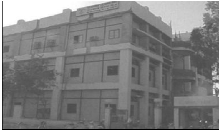
Figure 81: A partial collapse of the burnt-clay brick masonry infill held together with cement mortar occurred in the upper story of a three-story telephone exchange building in Bhuj. The solution to this problem involved replacing the infills in the entire building with lightweight foam concrete panels. The new panels were placed between asbestos sheets and secured to the building's frame using thin steel straps, including those at the lower stories
