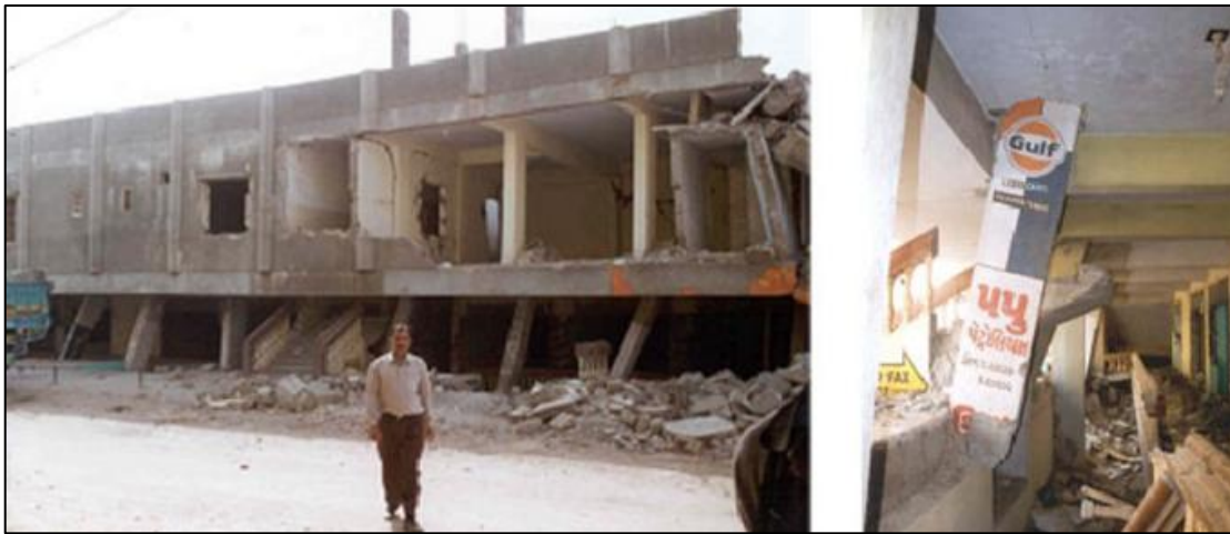
Figure 54: Image showing collapsed apartment complex in Gujarat, due to lack of continuous reinforcement causing failure where in, columns failed to resist shear and moments due to poor detailing and materials, particularly at the top and bottom of the columns. The basement and first storey levels collapsed, and the columns punched through the slab after shearing off the beam-column connection.
