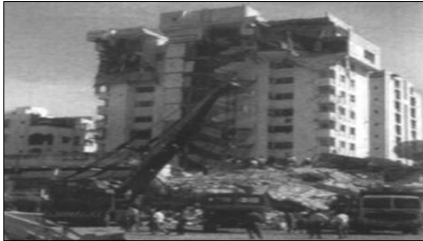
Figure 65: Collapse of flexible side of 11-story apartment building in Ahmedabad due to plan Irregularity
