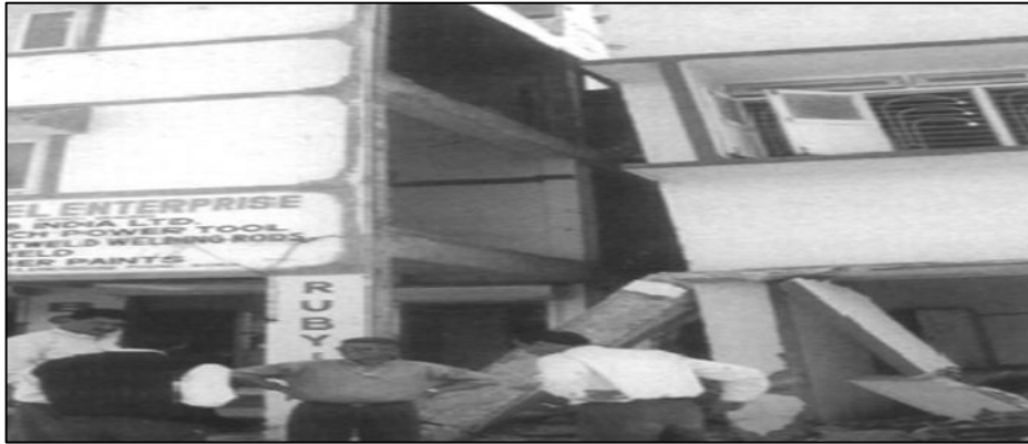
Figure 56: This area of Gandhidham has many row constructions where there is little to no space between adjoining buildings. In some cases, infills are only made in one of the two buildings at the interface. The building on the left had no infills in the upper stories, while the building on the right experienced a collapse at the ground story.
