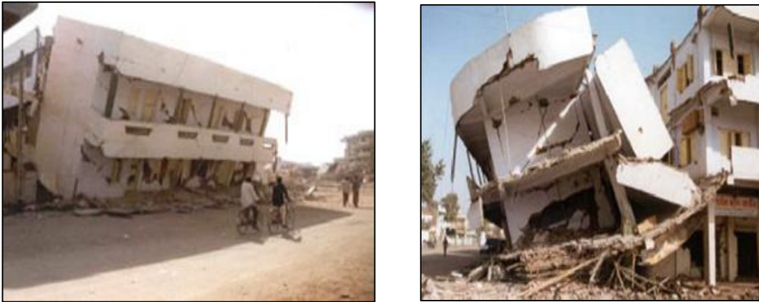
Figure 53: Image showing soft storey building collapse in Gandhidham, highlighting absence of structural integrity.
