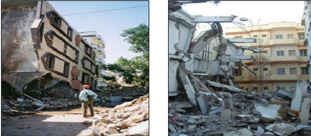
Figure 41: Overturned building in Bhuj
