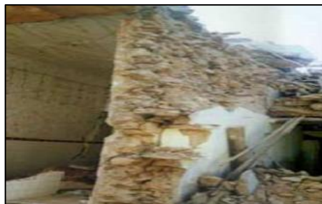
Figure 32: Damage to a rubble stone and mud mortar house in old Bhuj
