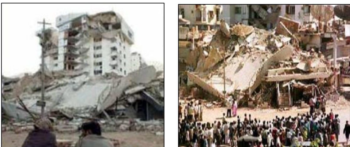
Figure 61: The multistorey building (Mansi complex) in Ahmadabad soon after the earthquake, shown in both general and close-up views.
