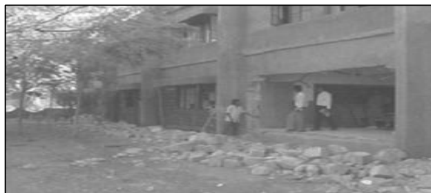
Figure 80: At a two-story school building in Ahmedabad, the large block sandstone masonry infills in cement mortar were replaced entirely with burnt-clay brick masonry infills in cement mortar.
