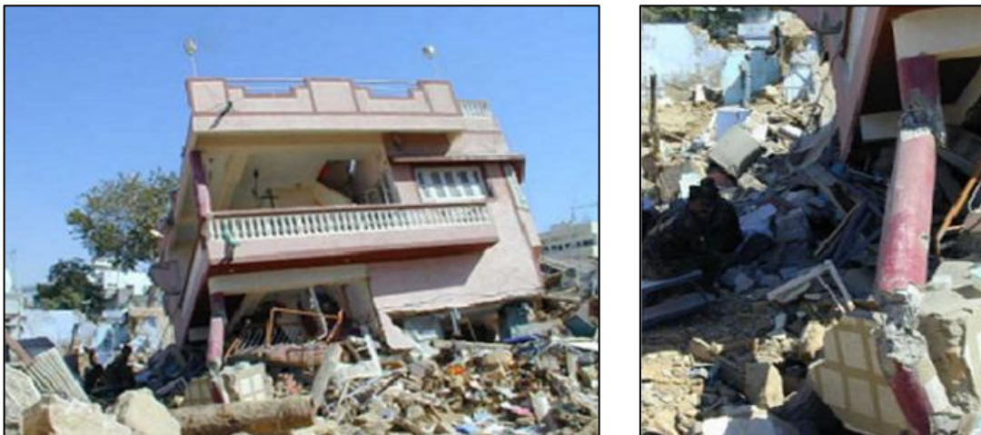
Figure 42: Building collapse in Bhuj
