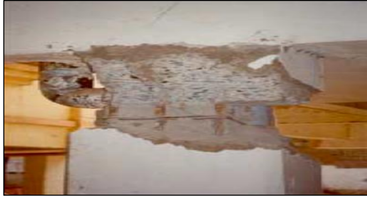
Figure 70: Ground floor column in Akshardeep apartment complex, Ahmadabad
