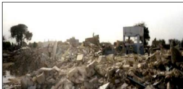
Figure 13: Destruction of masonry structures in the old section of Anjar
