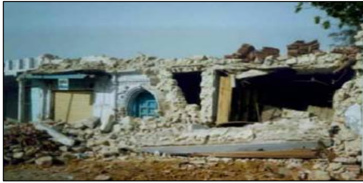
Figure 33: Damage to cutstone and lime mortar masonry building in old bhuj
