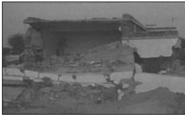
Figure 27: Collapse of this masonry structure was done to wall failure
