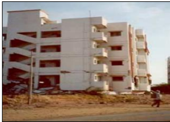
Figure 38: Soft storey collapse of a five storey apartment building in Bhuj
