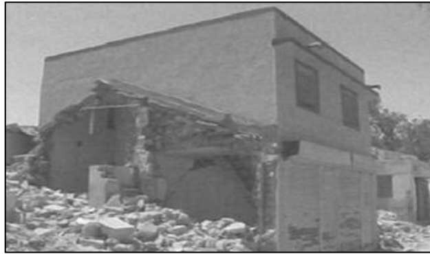
Figure 19: The inclined concrete stair slabs may have added lateral strength to weak masonry.
