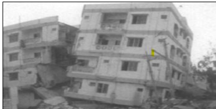
Figure 47: collapse of a partially open ground story building in bhuj , coupled with vertical split of the building at the midline
