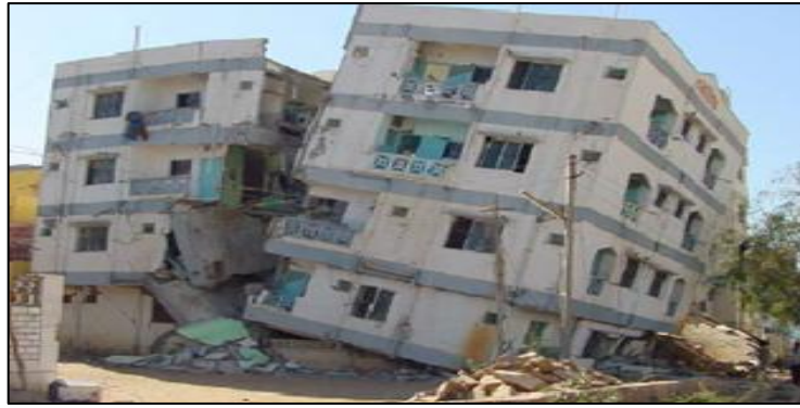
Figure 45: Collapsed open ground storey building in BHUJ
