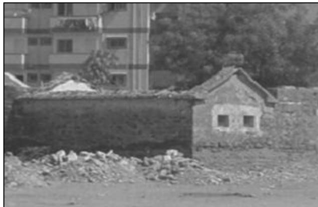
Figure 28: In a few instances, such as this masonry structure, the roof alone was responsible for Structural collapse
