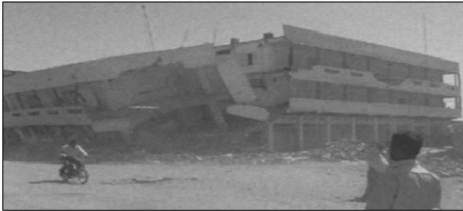
Figure 59: collapse of a corner of an L-shaped building in Gandhidham was caused by the failure of the floor diaphragm at the re-entrant corner.
