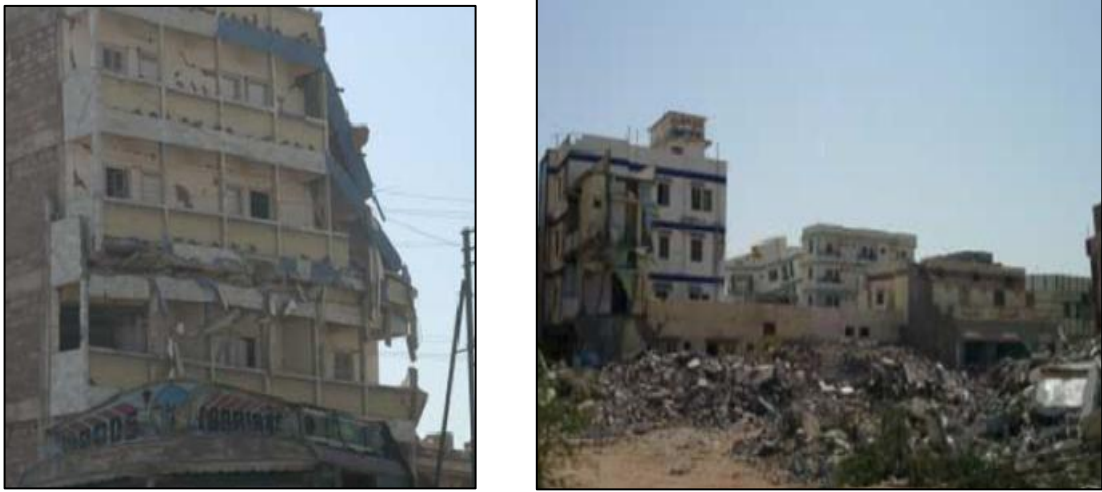
Figure 43: Partly collapsed massive concrete framed building structure with infill brick masonry wall
