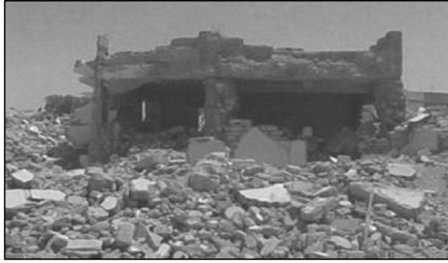
Figure 18: This building with post system survived in collapsed old Anjar
