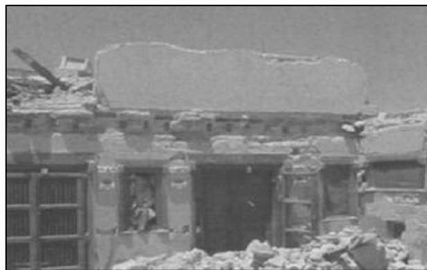
Figure 21: Floor separation occurred during intense shaking.
