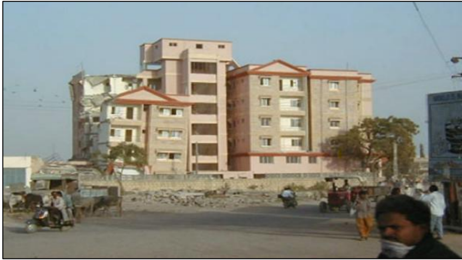
Figure 12: Partial collapse of an apartment building Anjar
