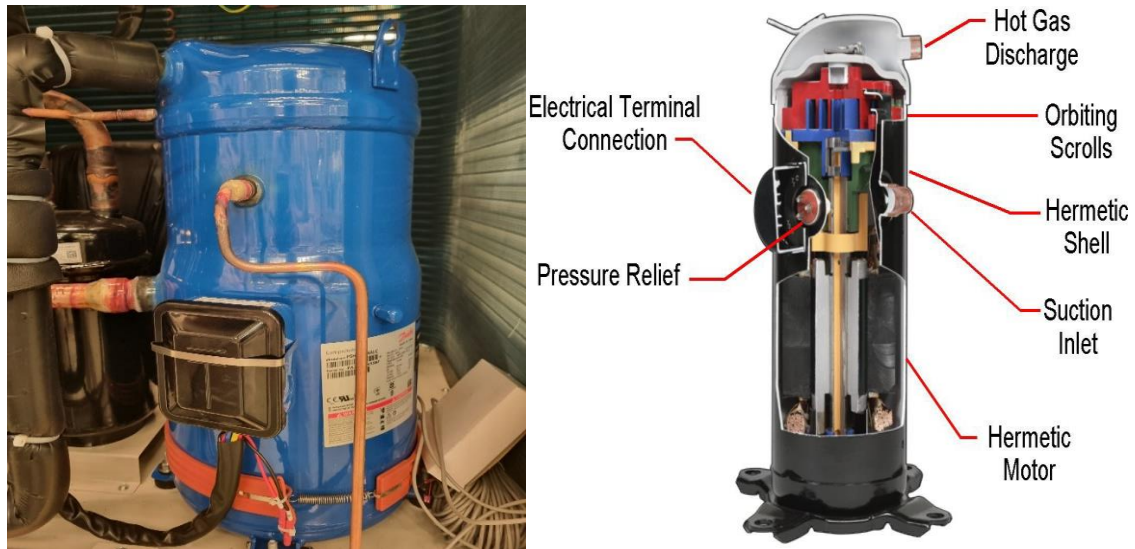
Figure 1.9.1 Scroll Compressor [19]
