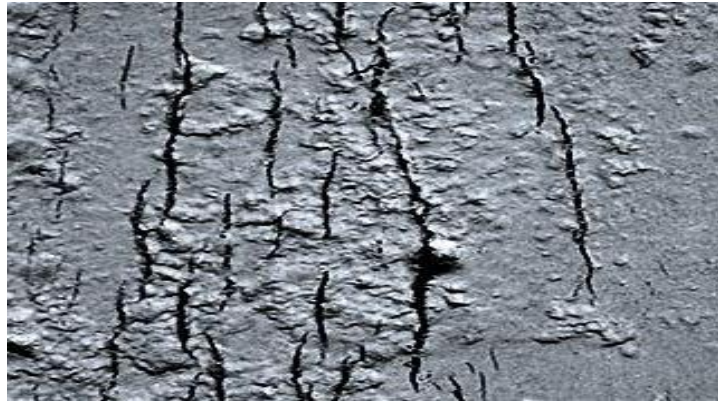
Figure 1.7: Colony of stress corrosion cracks
