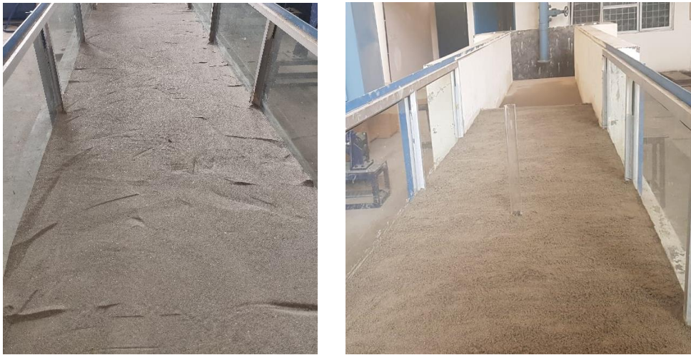
Fig. 3.9 (a) Placement of sand bed; (b) placement of the pier
