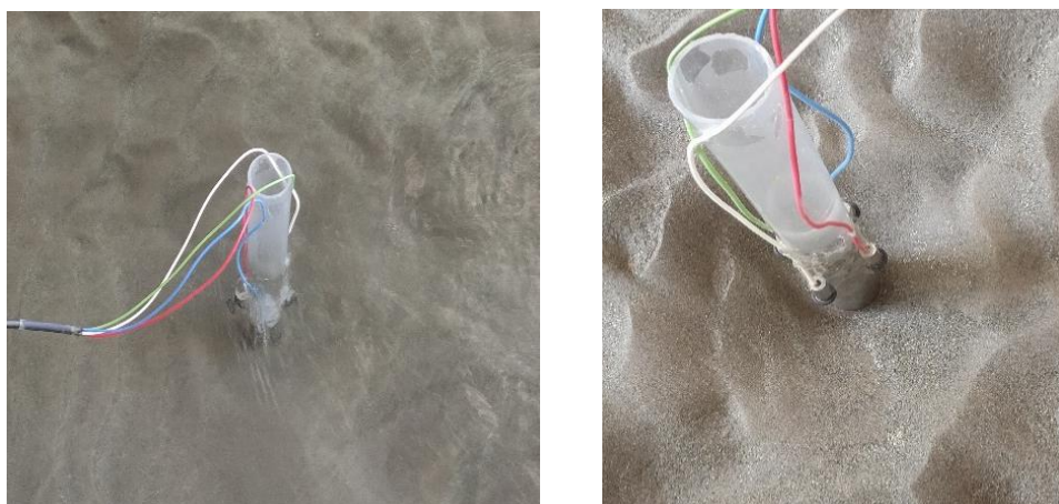
Fig. 3.10 Installation of SeaTek transducers around the pier
