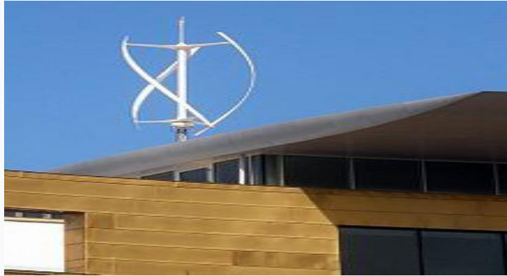
Fig.13. Small vertical wind turbine
