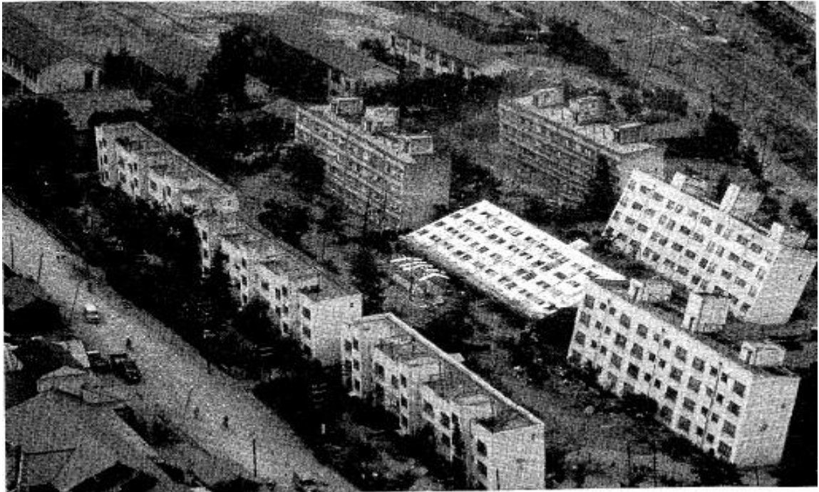
Figure 1.1 Bearing capacity failures cause due to liquefaction of the Kawagishi-cho apartment building following the 1964 Niigata earthquake.
