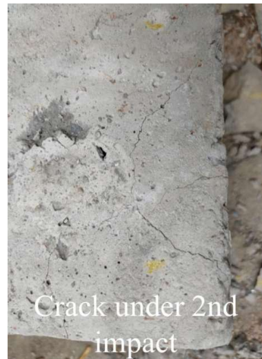
Figure 4.26 Progress of crack in 2 nd impact
