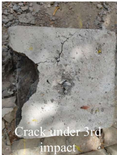
Figure 4.25. Cracks under third impact
