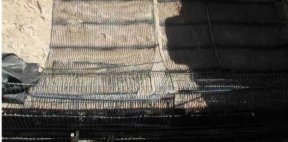
Figure 3.4 Photo of GRS extensible reinforcement (geogrids)
