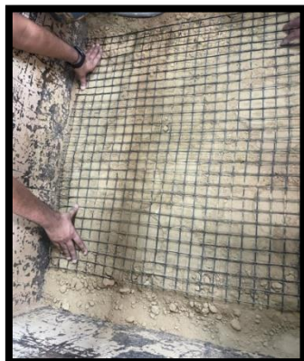
Fig.4.3 Laying of geogrid layer
